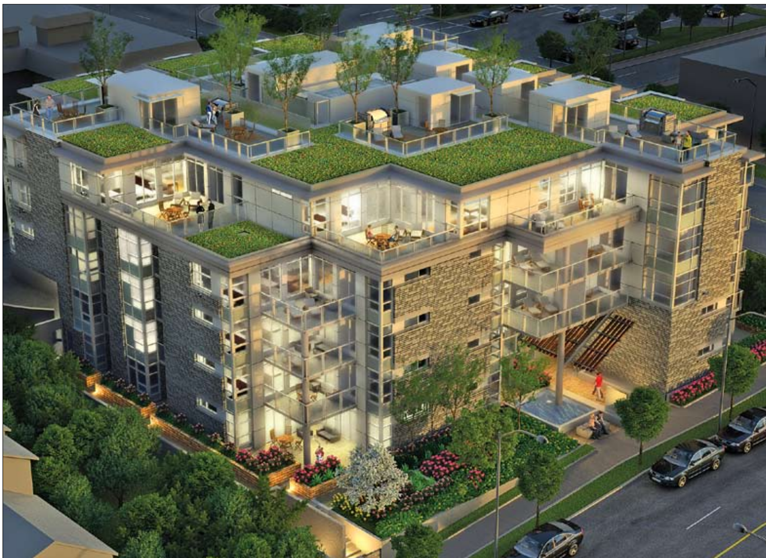
CONTINUED ON P.6 Waterfront Capital Partners’ The Kimpton in North Vancouver offers brand-new condo homes that feature a sustainable green roof.
