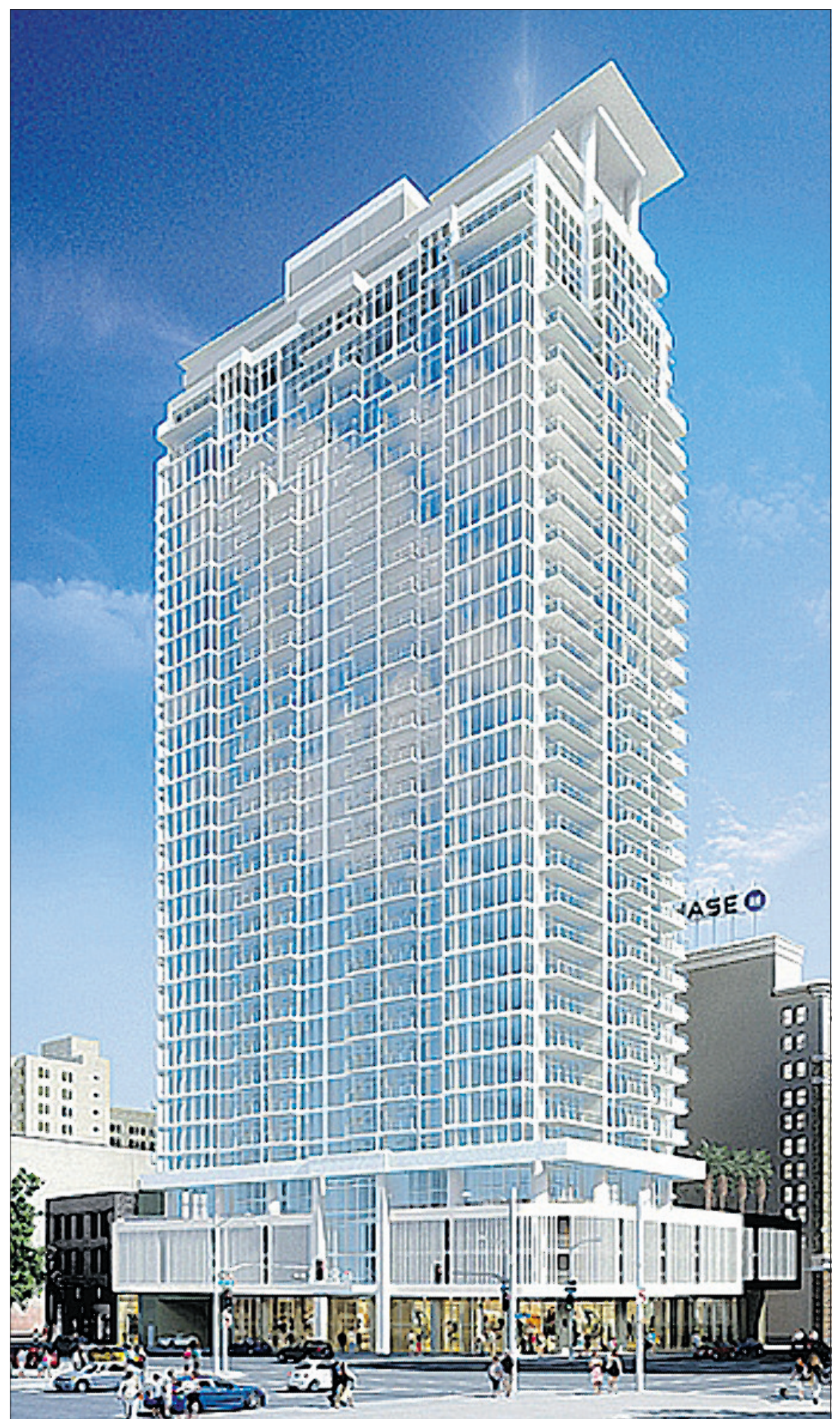
A 32-storey highrise under construction in downtown L.A. will include 283 luxury apartments.
